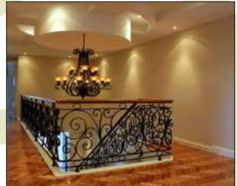
Wrought-Iron Lace Work, w' Timber Handrail
