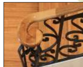
Handrail Starting Scrolls
