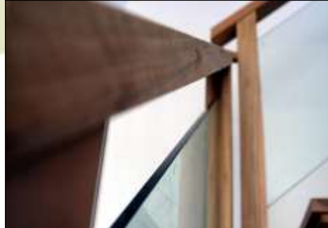
Glass - w' Timber Support Posts
