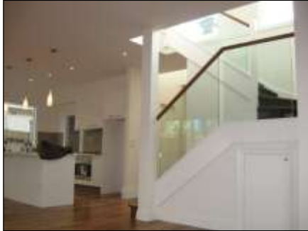
Glass (12mm Toughened) - Inserted into Staircase String
